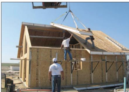
**NetSolar Construction workers piece together the structural insulated panels of a home. The panels create a tight exterior envelope, making them green and energy efficient.**
